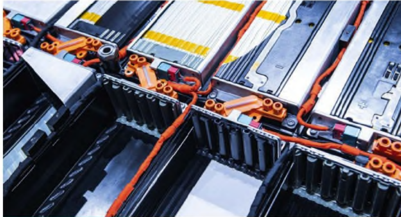
For electric powertrains, keeping the battery modules cool is crucial to ensuring optimum performance
